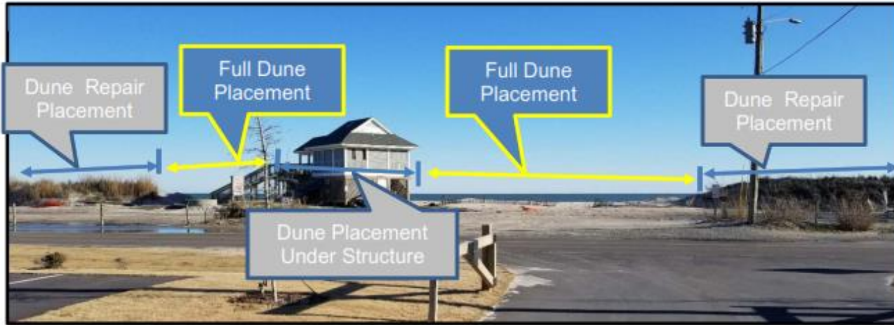
Figure 1: Dune Material Placement (photo taken February 3, 2021).
