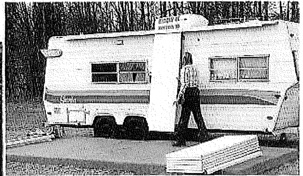
2. Roof panel slides easily into adapter rail.
